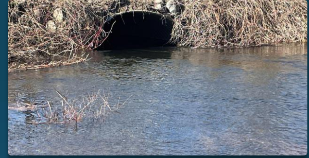
Bridge St. Culvert Ellsworth
