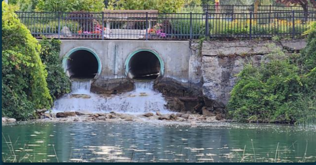
Elk Rapids Overflow Spillway
